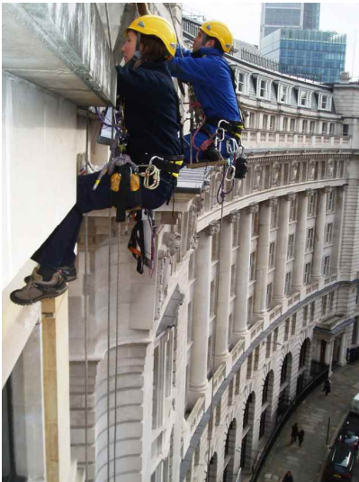
GPR can be used successfully to investigate listed buildings where minimal disturbance to the fabric of the structure is of paramount importance.
