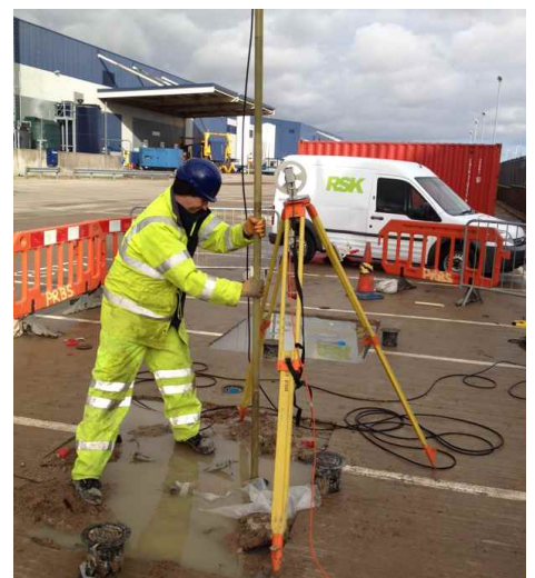
A Borehole GPR probe being lowered into the hole.
