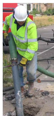
Hydro-vac excavation can be used to safely expose buried live utilities.
