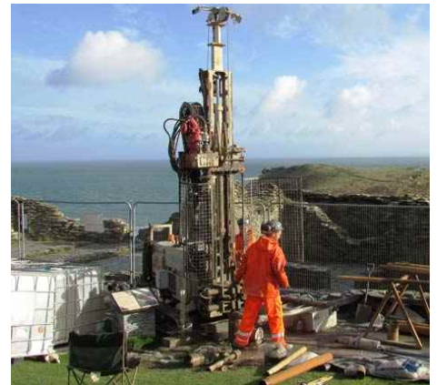
Borehole geophysics requires the use of an existing or newly prepared borehole or array of boreholes in order to carry out the testing. RSK can provide borehole drilling and installation services as part of the overall testing package.
