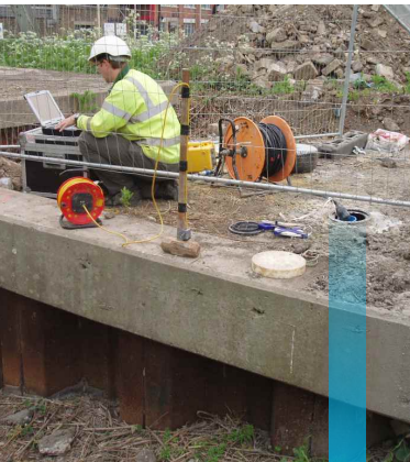
The parallel seismic method being used within an adjacent borehole to ascertain information on the depth of a sheet pile. Note access to the top of the pile is required.
